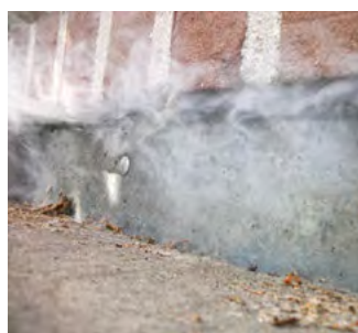
Evidence of defective sealing of the wall connection above an underground garage.
