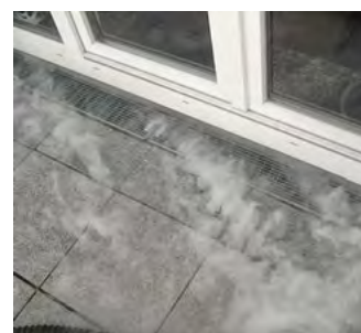
Defective sealing of a roof-top terrace.
